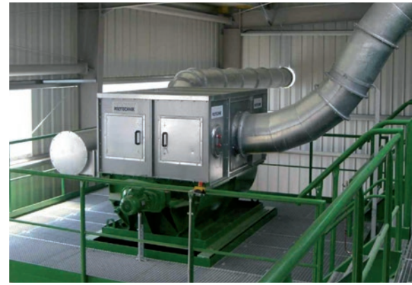
Separator PMA with sound insulation for housing
