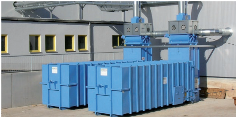
Separator PMA with sound insulation for housing
