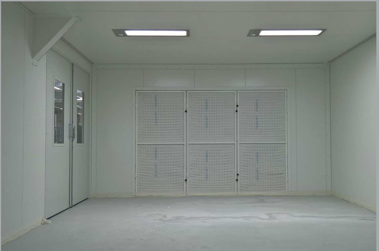
The exhaust area within the cabin allows for flexible operation.
