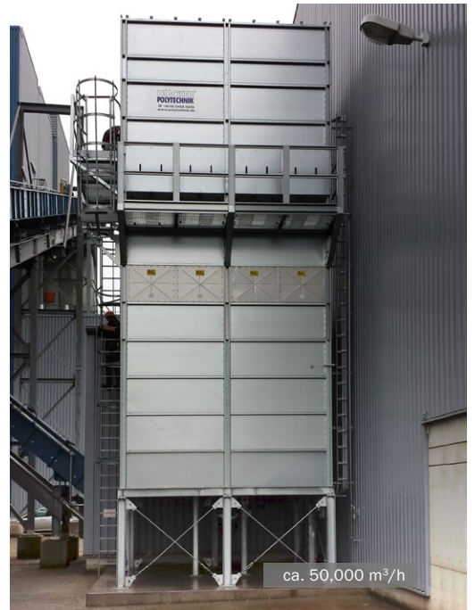
MultiStar stirrer device filter • biomass power plant
