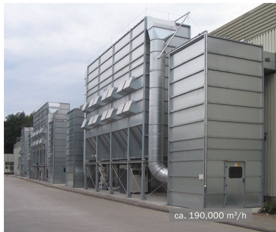
MultiStar reverse air flow filter • kitchen manufacturing
