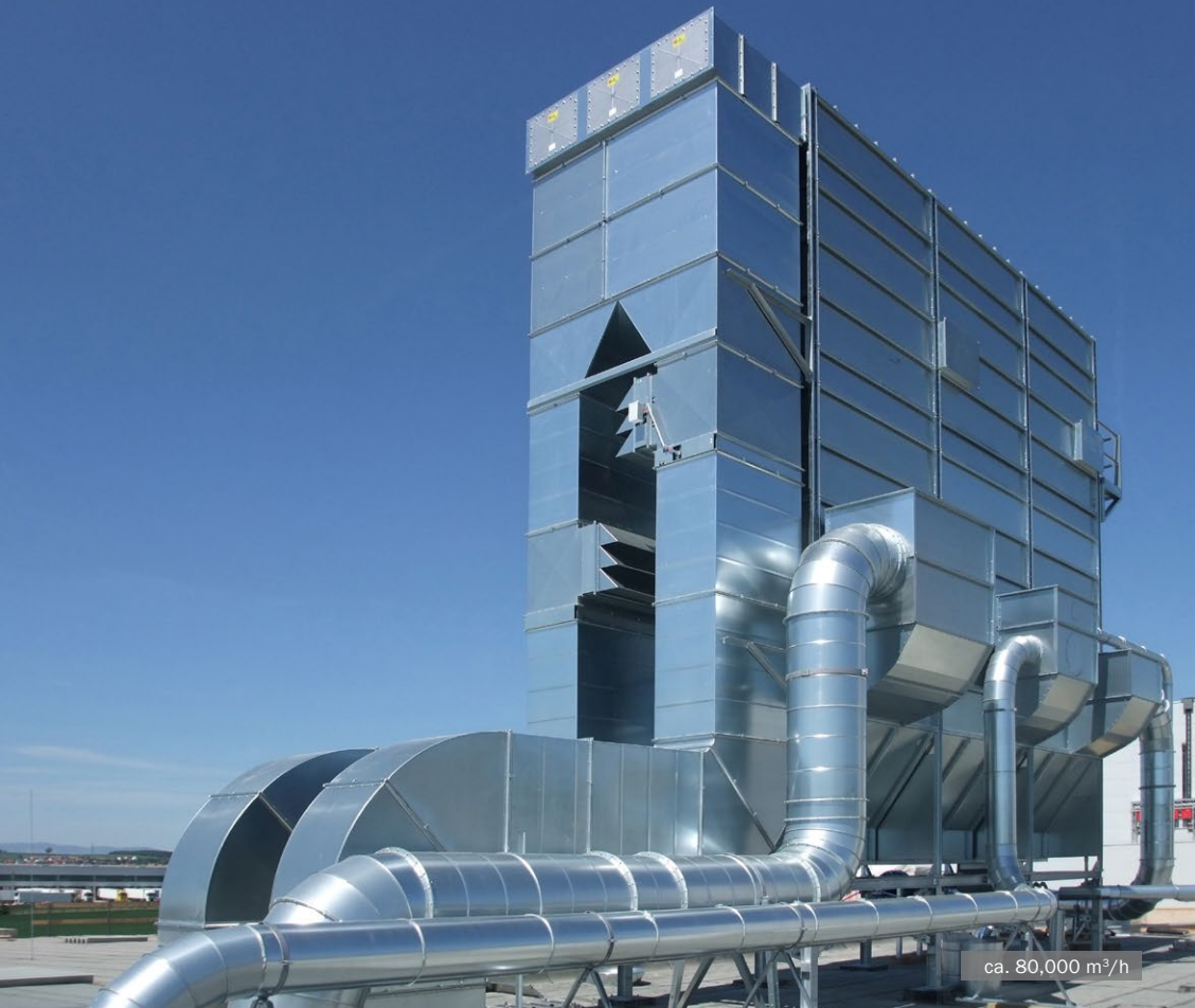
MultiStar screw filter with scavenging air cleaning • sport equipment production
