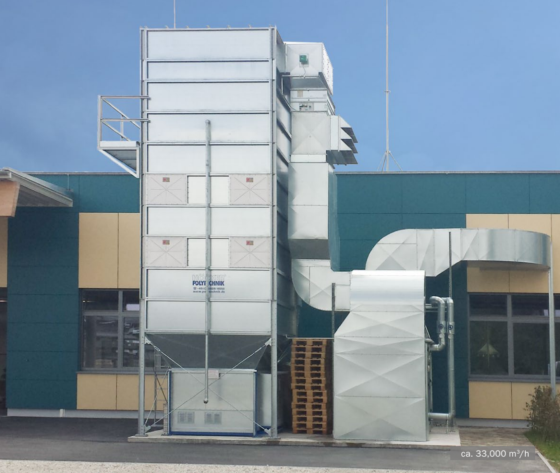
MultiStar with integrated briquetting press and heat recovery system • vocational school
