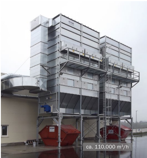
MultiStar screw filter with jet cleaning • interior work
