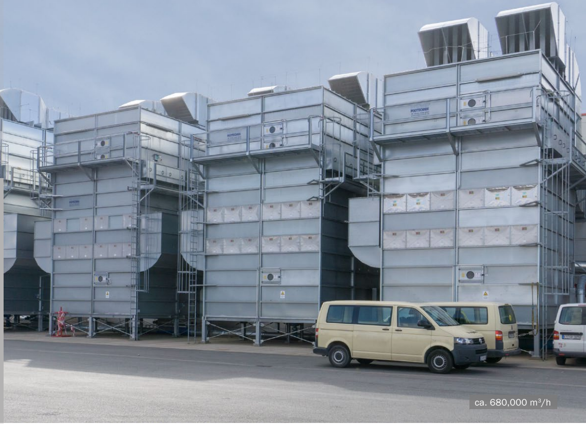
MultiStar stirrer device filter with jet cleaning • kitchen manufacturing
