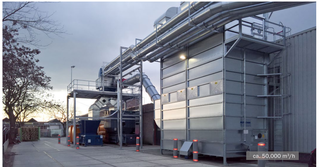
MultiStar sliding bar filter with jet cleaning • printing and packaging industry
