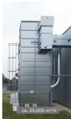
MultiStar press filter • interior work
