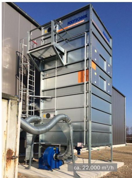
MultiStar stirrer device filter • laminated beams production
